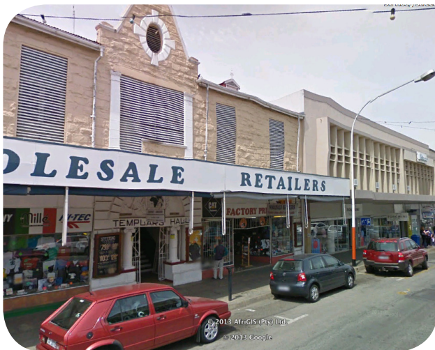
FIG.1.52 THE DEGRADATION OF HISTORIC BUILDING FACADES IS TAKING PLACE IN THE HISTORIC CENTRE OF OUDTSHOORN
