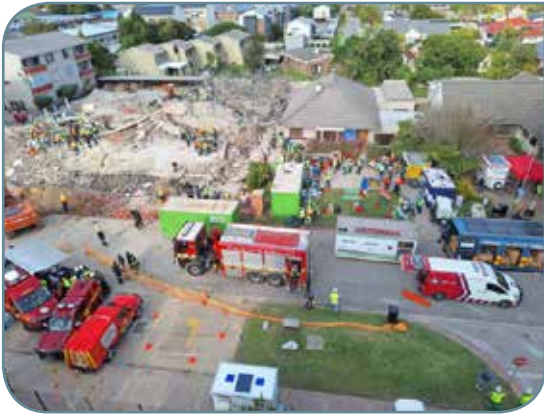
Figure 32: Shortly after the building collapsed
