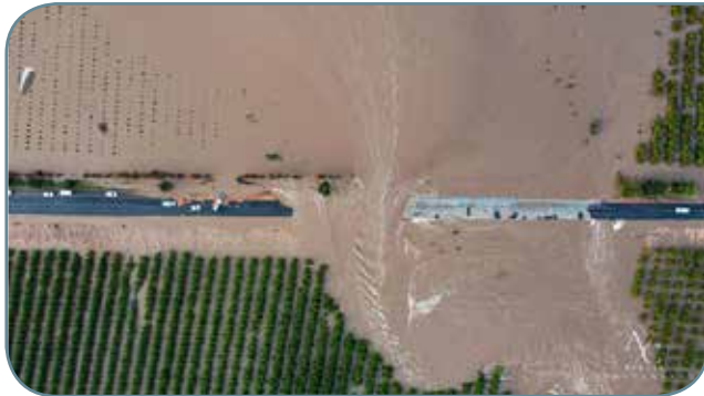
Figure 30: Major road damage to the entrance of Citrusdal
