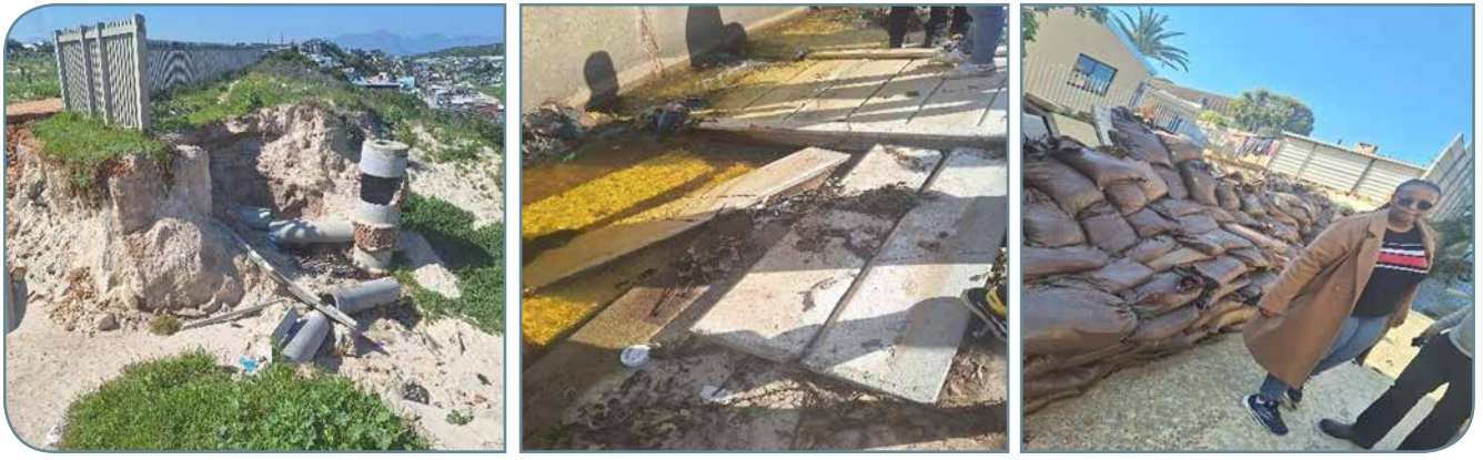
Figure 49: City of Cape Town damages
