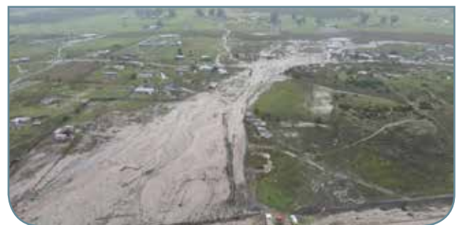
Figures 31: Damage caused by the multiple dam wall break in Riverlands, Swartland
