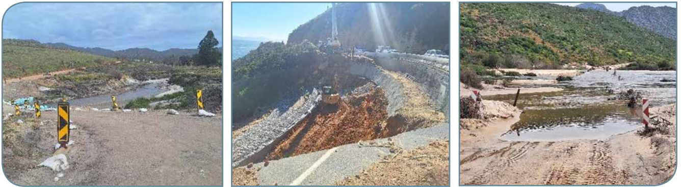
Figure 62: Department of Infrastructure damages
