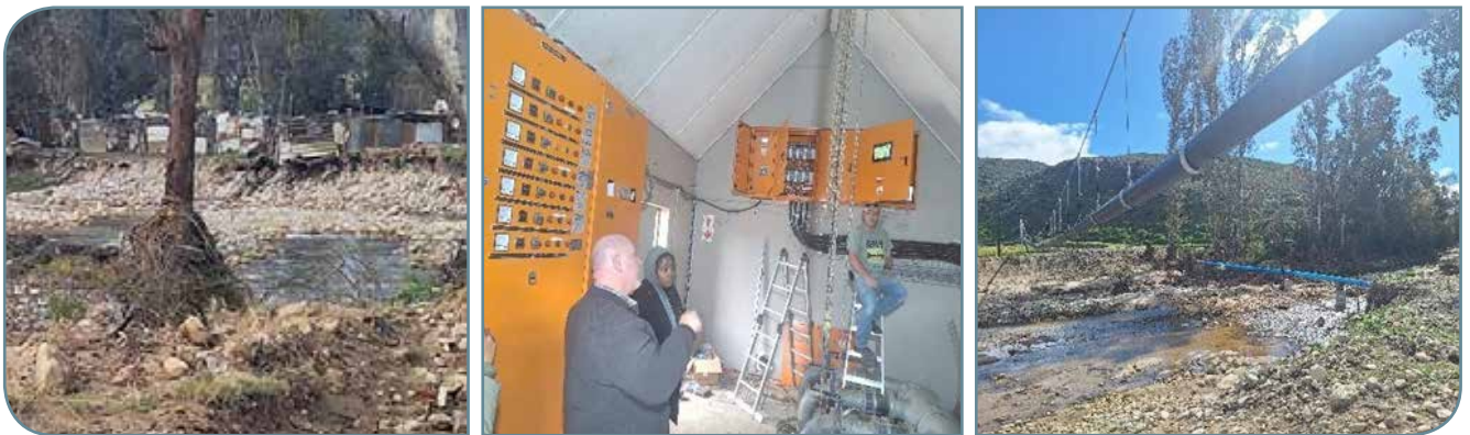
Figure 55: Langeberg Municipality damages
